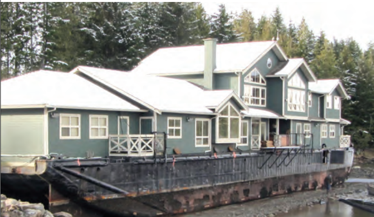
The "Big Time Sportfishing Resort" on its deteriorating steel barge.
