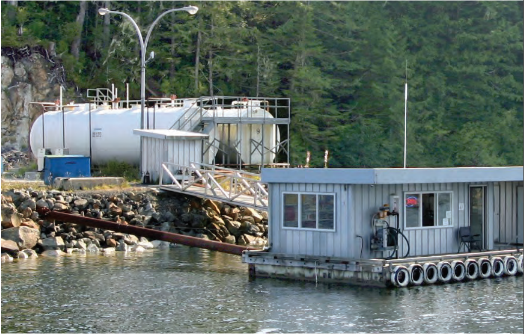
The floating concrete fuel station was designed and constructed entirely in Shearwater's shop in 2000 and launched with the 70-ton travel lift. Equipped with the latest fuel equipment and metering, the station had an office, sales area, breezeway, two bathrooms and a product storage room atop a 1,200-square-foot float.
